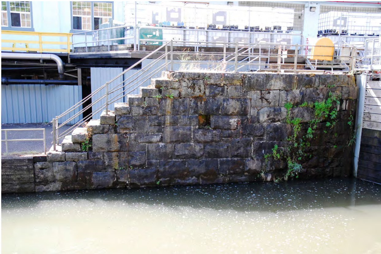
Figure 9: View of Ashlar Masonry at Gate 4, Mill Side
