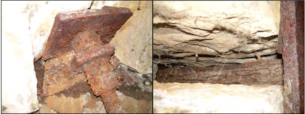
Figure 13: View of gudgeon anchor rod at Gate 4, Mill Side
